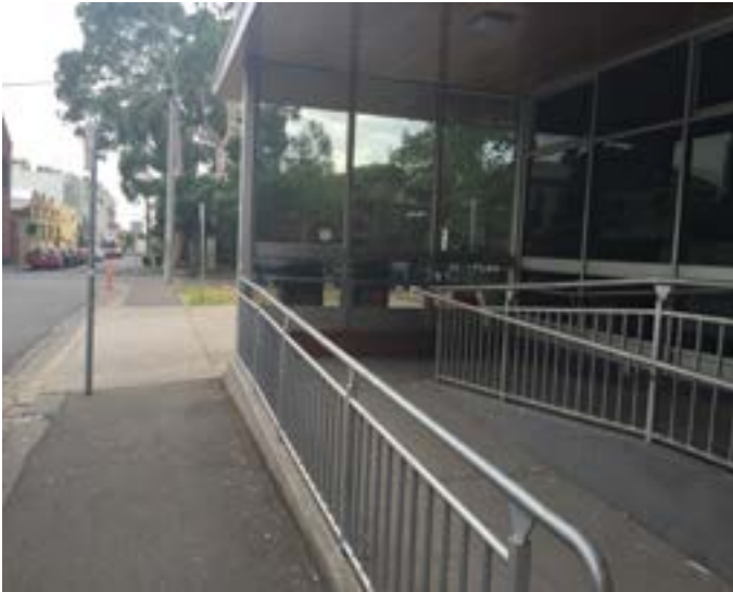
Moor St entrance
