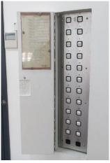
Three banks of dimmable house lights can be controlled from the control room. The dimming faders are located on the wall to the left of the window. The switch labelled DIMMERS must be turned on. The switches on the rear wall of the control room, above the fuse box labelled DMR LIGHT CONTROL must also be switched on.
